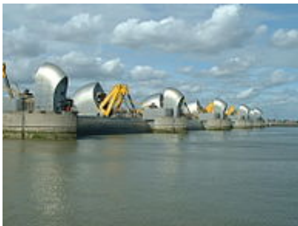
The flood barrier on the river Thames near London, England Source: Andy Roberts - Flickr.com, https://commons.wikimedia.org/w/index.php?curid=341229
